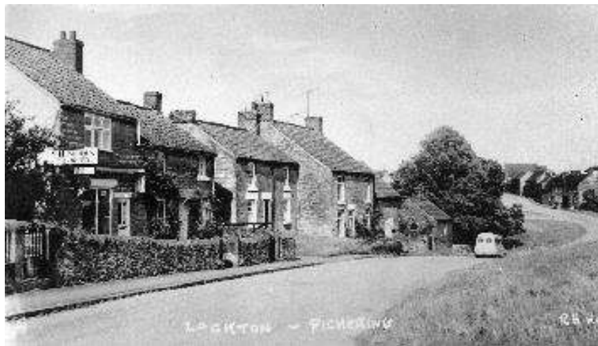
37. The thatched cottage rebuilt as Mrs Burden's grocers shop.
