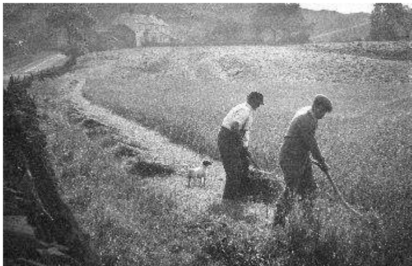
12. Tom and Edwin Warriner 'opening-up' a field of corn ready for the binder. The photograph was taken in 1944, Saltergate Inn and Bank are in the background
