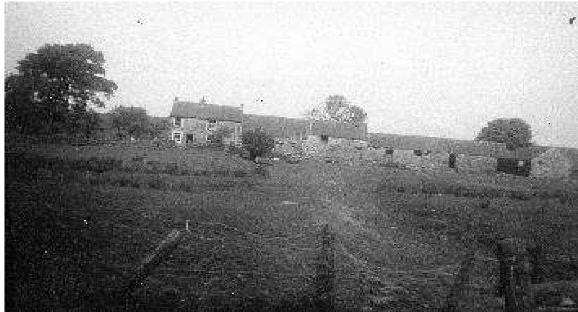
16. Whinny Nab Farm, now demolished.
